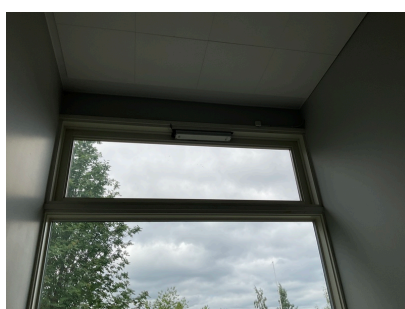
Smoke extraction window for building A and building B
