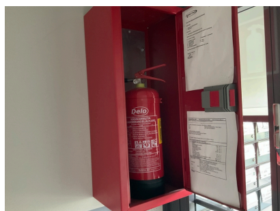
6kg ABC Dry Powder portable fire extinguisher
