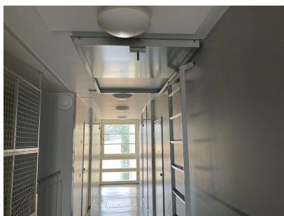
Building C access to ventilation
