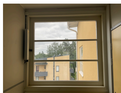
Smoke extraction window in building C
