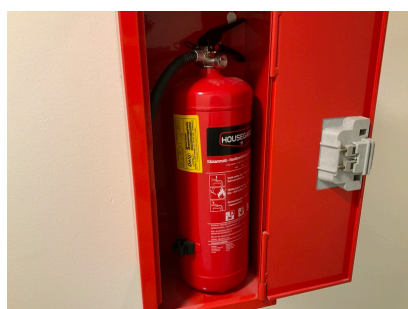
Entrance B 6kg ABC Dry Powder portable fire extinguisher
