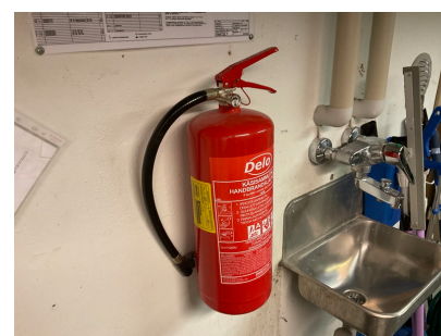
Heat distribution room fire extinguisher 6kg ABC Dry Powder
