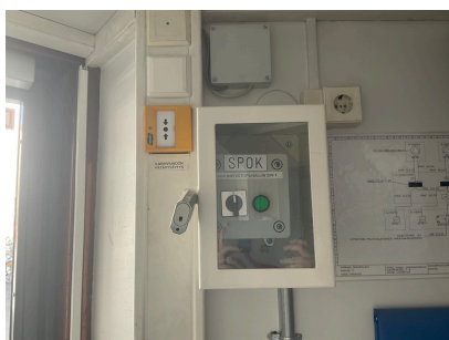
Smoke extraction fan activation and emergency shut-off button for ventilation
