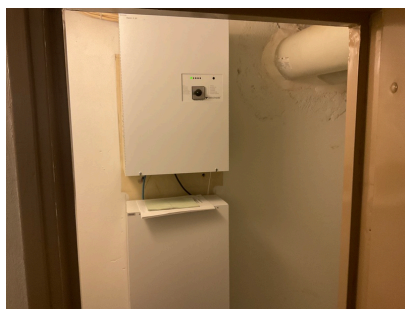
Safety lighting control panel in the basement corridor
