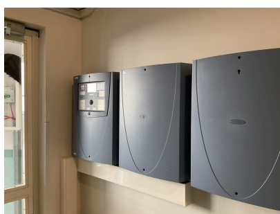
Fire alarm system control panel on the ground floor of entrance B, on the side of the inner yard
