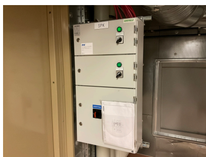
Smoke extraction system control panel in the ventilation machine room
