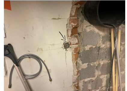
Pipe lock in the heat distribution room
