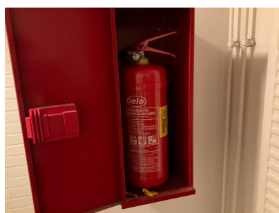
Portable 6kg ABC Dry Powder fire extinguisher
