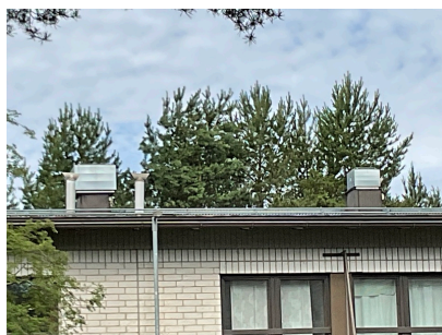
Roof ventilation ducts
