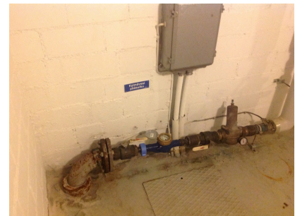
Main water stopcock in staircase D
