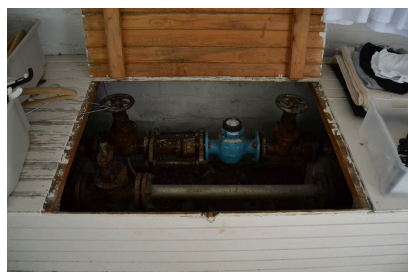
Main water stopcock, encased
