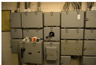
The apparatus of the main electrical switchboard
