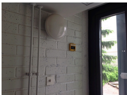
Air-conditioning emergency stop at the entrances on the side of the inner courtyard
