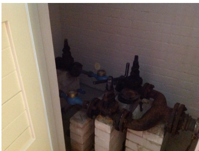
Main water stopcock in basement A
