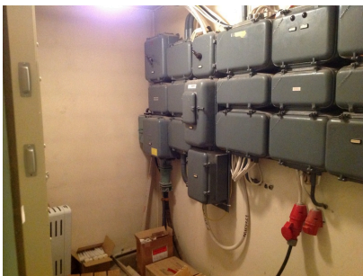
Main electrical switchboard in the basement corridor
