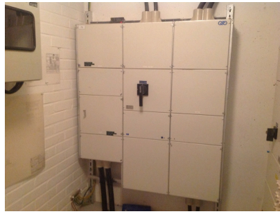
Main electrical switchboard in basement DE
