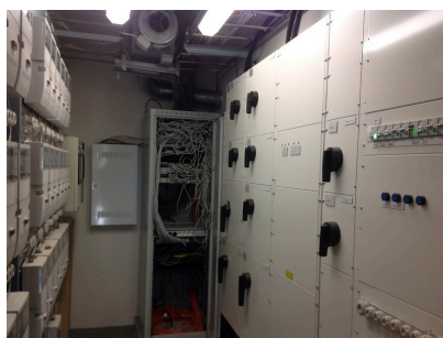
Main electrical switchboard in building B
