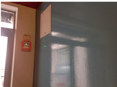
Air-conditioning emergency stop and smoke extraction activation switches at the entrances
