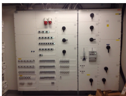
Main electrical switchboard in basement C
