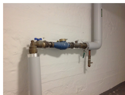
Main water stopcock in basement C
