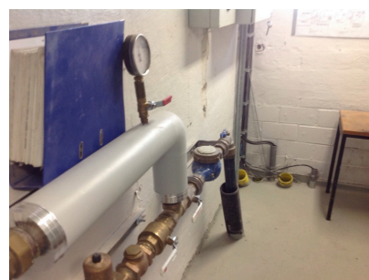
The main water stopcocks in the heat distribution rooms
