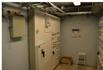
The apparatus of the main electrical switchboard
