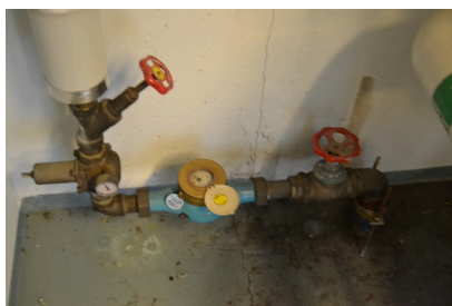
Main water cut-off valve
