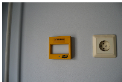
Air-conditioning emergency stop button
