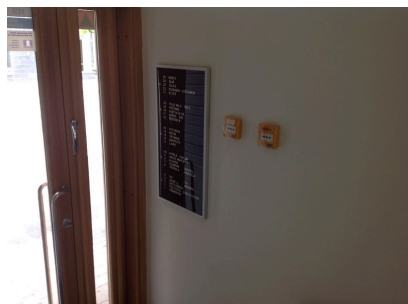
Air-conditioning emergency stop and smoke extraction activation switches at the entrance
