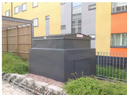
The smoke extraction hatch of the parking garage in the inner courtyard
