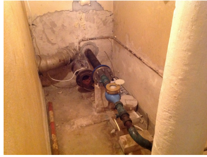
Main water cut-off valve in the basement
