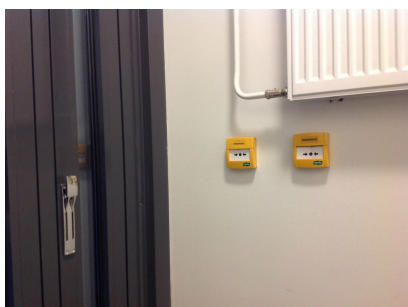
Smoke extraction activation and air-conditioning emergency stop at the entrance
