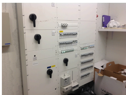
Electricity switchboard
