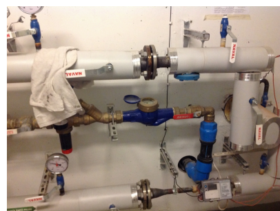
The main water cut-off valve in the heat distribution room
