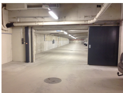
Automatic fire door in the parking garage
