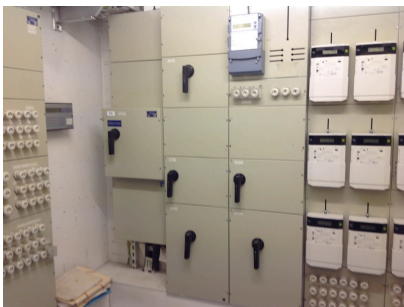
Electricity switchboard
