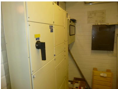
Electricity switchboard
