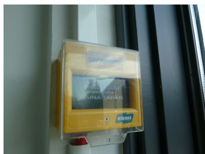
Manual smoke extraction activation
