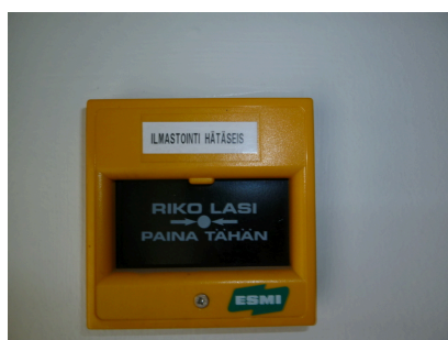
Air-conditioning emergency stop
