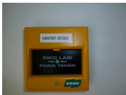
Air-conditioning emergency stop
