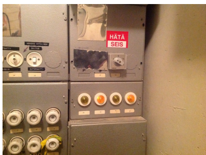
Air-conditioning cut-off
