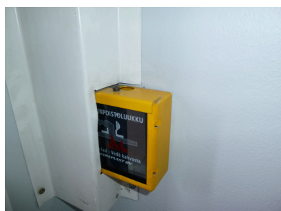
Manual smoke extraction activation
