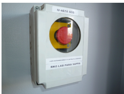
Air-conditioning emergency stop
