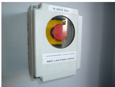
Air-conditioning emergency stop
