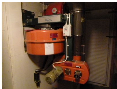
The air-conditioning apparatus of civil defence shelter 2
