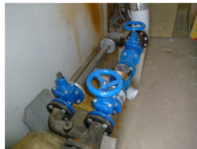
Main water stopcock, on the right side of the entrance of Tarmonkatu 6, staircase A
