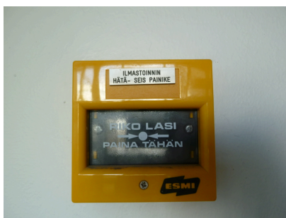
Air-conditioning emergency stop
