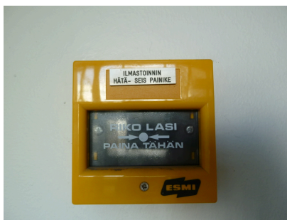
Air-conditioning emergency stop
