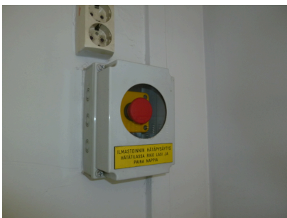
Air-conditioning emergency stop
