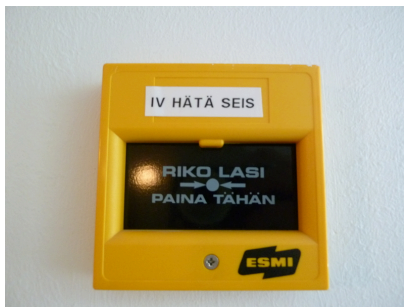
Air-conditioning emergency stop
