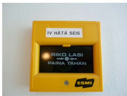
Air-conditioning emergency stop
