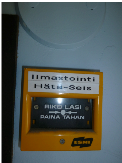
Air-conditioning emergency stop
