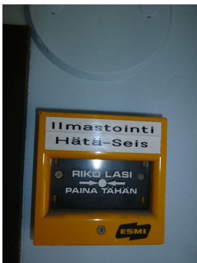
Air-conditioning emergency stop
