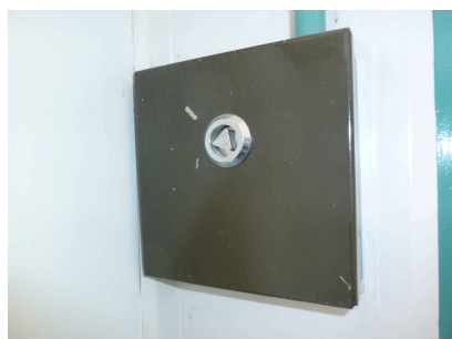
Manual smoke extraction activation
