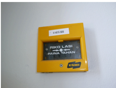
Air-conditioning emergency stop
