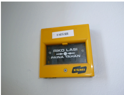
Air-conditioning emergency stop
