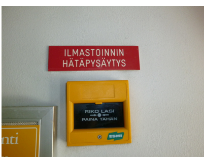
Air-conditioning emergency stop
