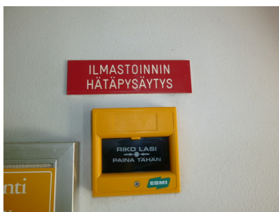
Air-conditioning emergency stop
