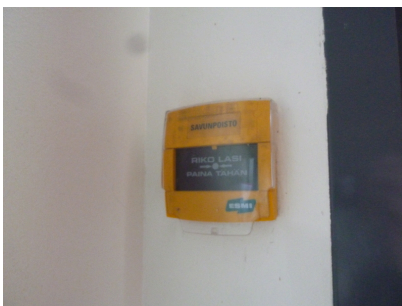
Manual smoke extraction activation
