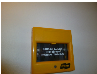
Air-conditioning emergency stop
