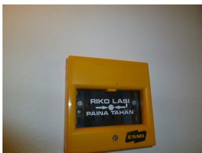
Air-conditioning emergency stop
