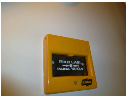
Air-conditioning emergency stop
