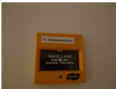
Air-conditioning emergency stop
