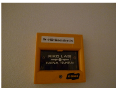
Air-conditioning emergency stop
