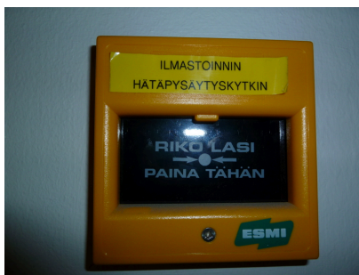
Air-conditioning emergency stop
