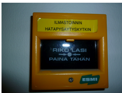
Air-conditioning emergency stop
