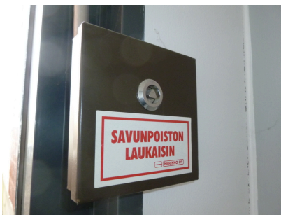
Manual smoke extraction activation
