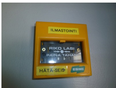
Air-conditioning emergency stop
