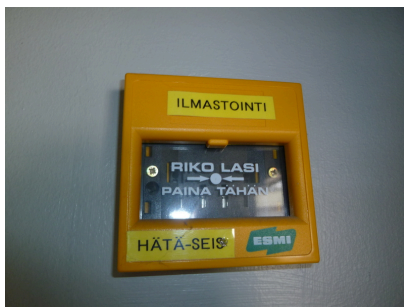
Air-conditioning emergency stop
