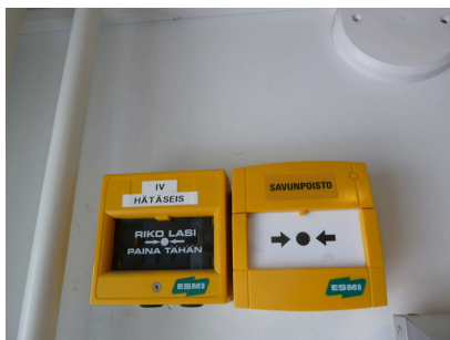
Air-conditioning emergency stop
