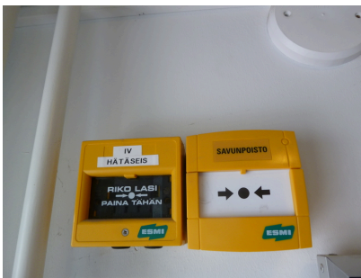
Air-conditioning emergency stop
