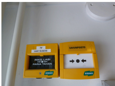
Manual smoke extraction activation
