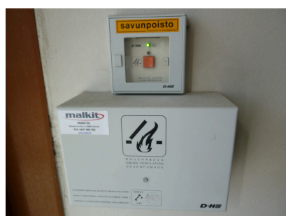
Manual smoke extraction activation
