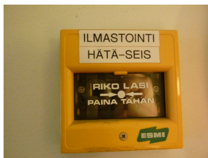
Air-conditioning emergency stop
