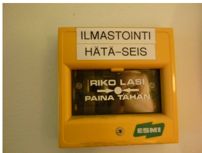
Air-conditioning emergency stop
