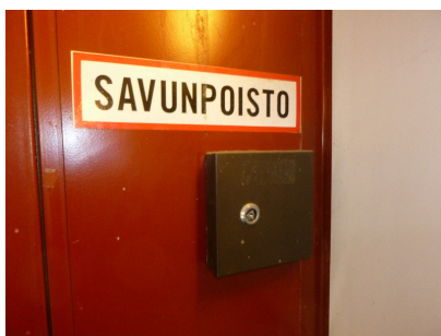
Manual smoke extraction activation
