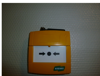
Air-conditioning emergency stop
