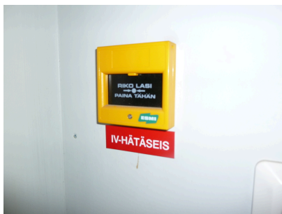
Air-conditioning emergency stop
