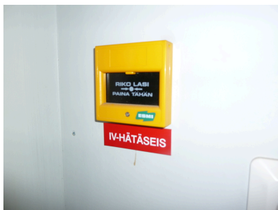
Air-conditioning emergency stop
