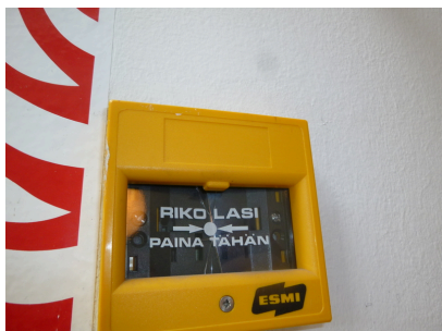
Air-conditioning emergency stop
