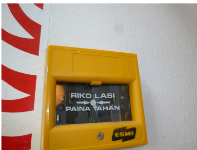
Air-conditioning emergency stop
