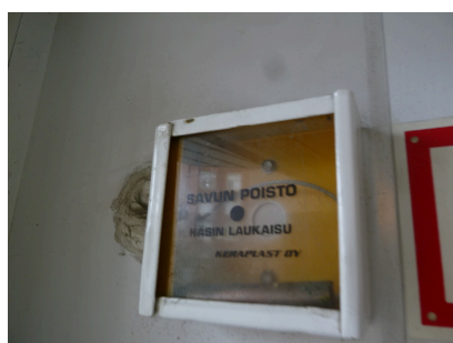
Manual smoke extraction activation
