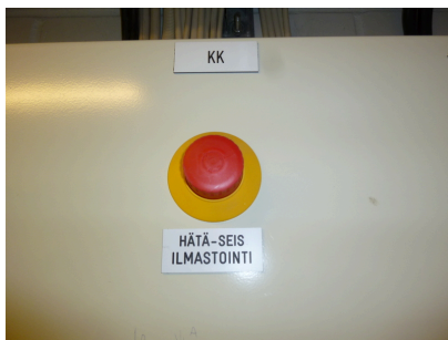
Air-conditioning emergency stop
