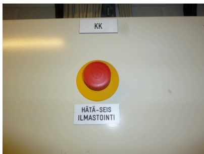
Air-conditioning emergency stop
