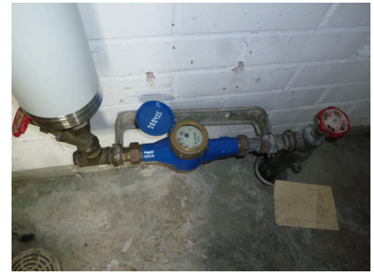
The main water stopcock of building C
