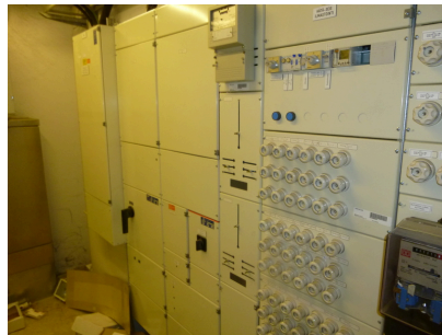
The main electrical switchboard of building A
