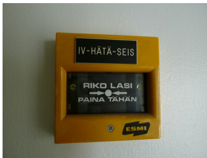
Air-conditioning emergency stop
