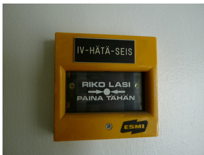
Air-conditioning emergency stop
