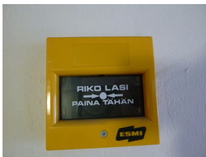
Air-conditioning emergency stop
