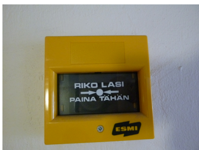
Air-conditioning emergency stop
