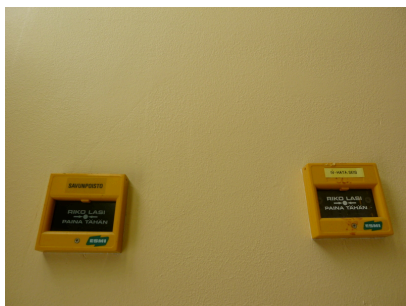
Manual smoke extraction activation
