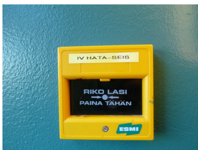
Air-conditioning emergency stop
