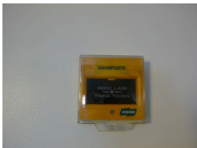
Manual smoke extraction activation
