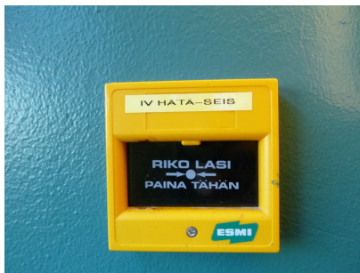
Air-conditioning emergency stop
