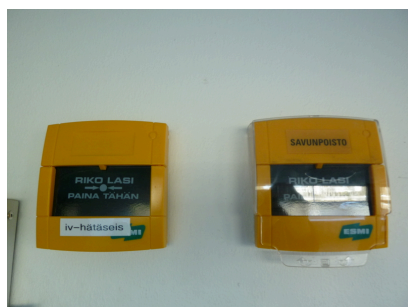
Air-conditioning emergency stop
