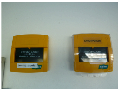
Air-conditioning emergency stop
