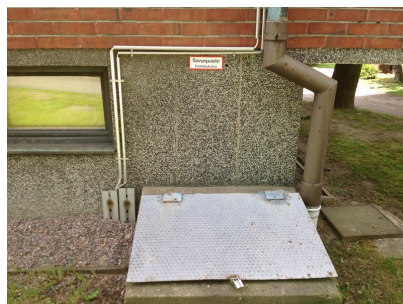
Smoke extraction of the civil defence shelter by opening the hatch
